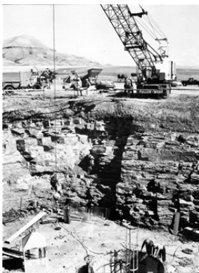
Early construction of a missile site
